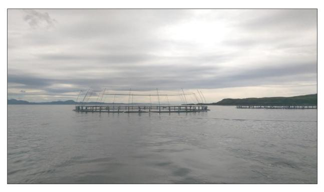
Figure 2: Typical pen design measuring 120m in circumference. This shows poles at the perimeter of the pen which support the top/bird netting and white pipes delivering the feed from the barge.
